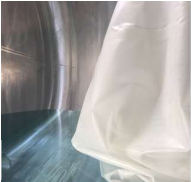
Outer steel shell tank with bladder inside, shown filling annulus with water
